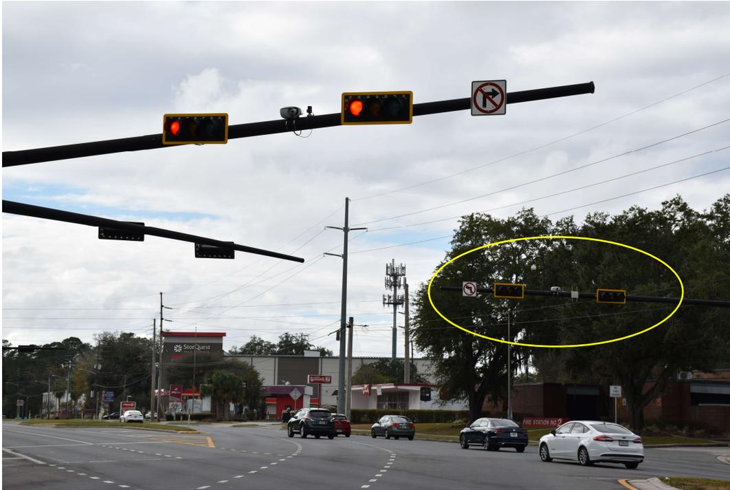
Figure 10. Right-side approach signal indications not visible to traffic on left-side approach
