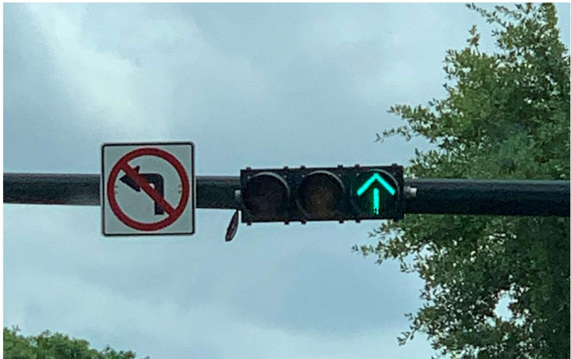
Figure 6. Vertical upward arrow to indicate straight-through movement
