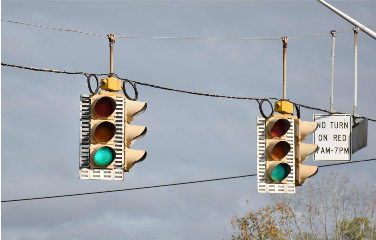
Figure 3. Faded paint on signal heads
