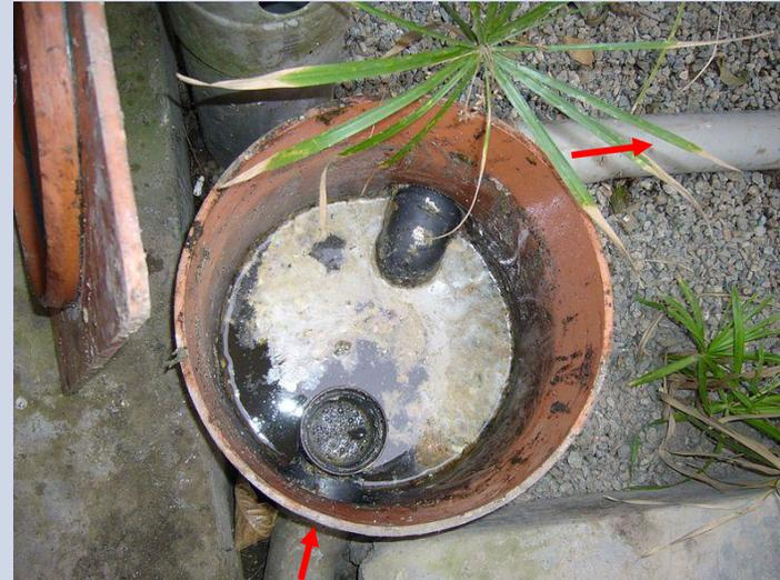
Figure 11: Examples of simple grease traps with flow direction arrows in red.
