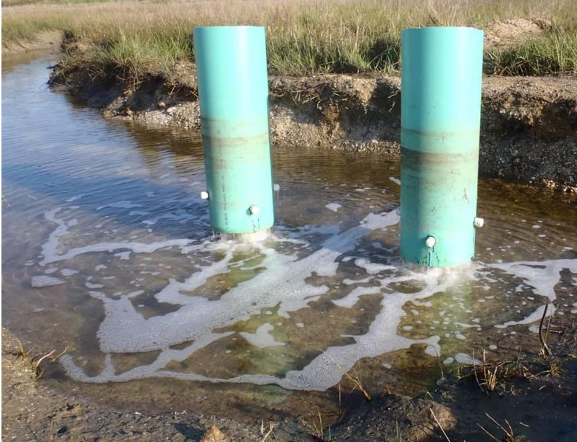
**Figure 10** – Two of the 4 Bi-directional Flow Pipes shown when discharging from the Pond into the Marsh. The brown stains indicate the various high tide elevations.
