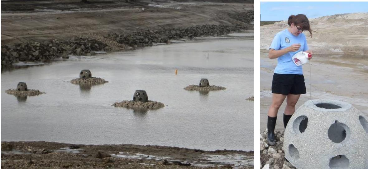
**Figure 16** – Some of the concrete Reef Balls located on the pond bottom during construction
