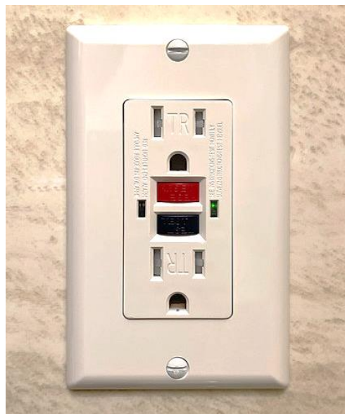
Figure 5: A typical residential GFCI receptacle in North America. The black button is labeled "test" and the red button is labeled "reset". The receptacle is labeled "TR" indicating tamper resistance.
