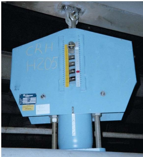
A typical Lisega constant support hanger: Its internal mechanism is completely different than other manufacturers. When reading the travel scale, it is typically in inches or mm, 0.25" in photo. As with other constant support manufacturers there is a red and white mark for the ambient and hot design locations.
