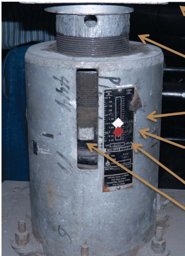
A typical variable spring floor support can and label
