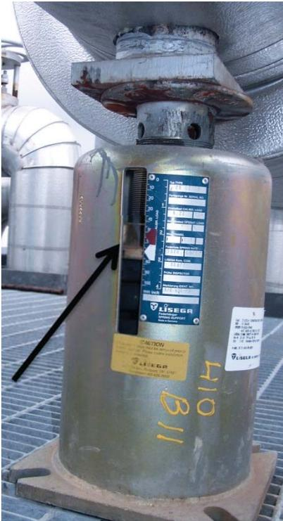
Lisega F style variable spring hanger. Scale has both inch and mm marks. There is no indicator tab. It should be read from the top of the load plate inside the can. In this case it is at 66mm or about 2-5/8".
