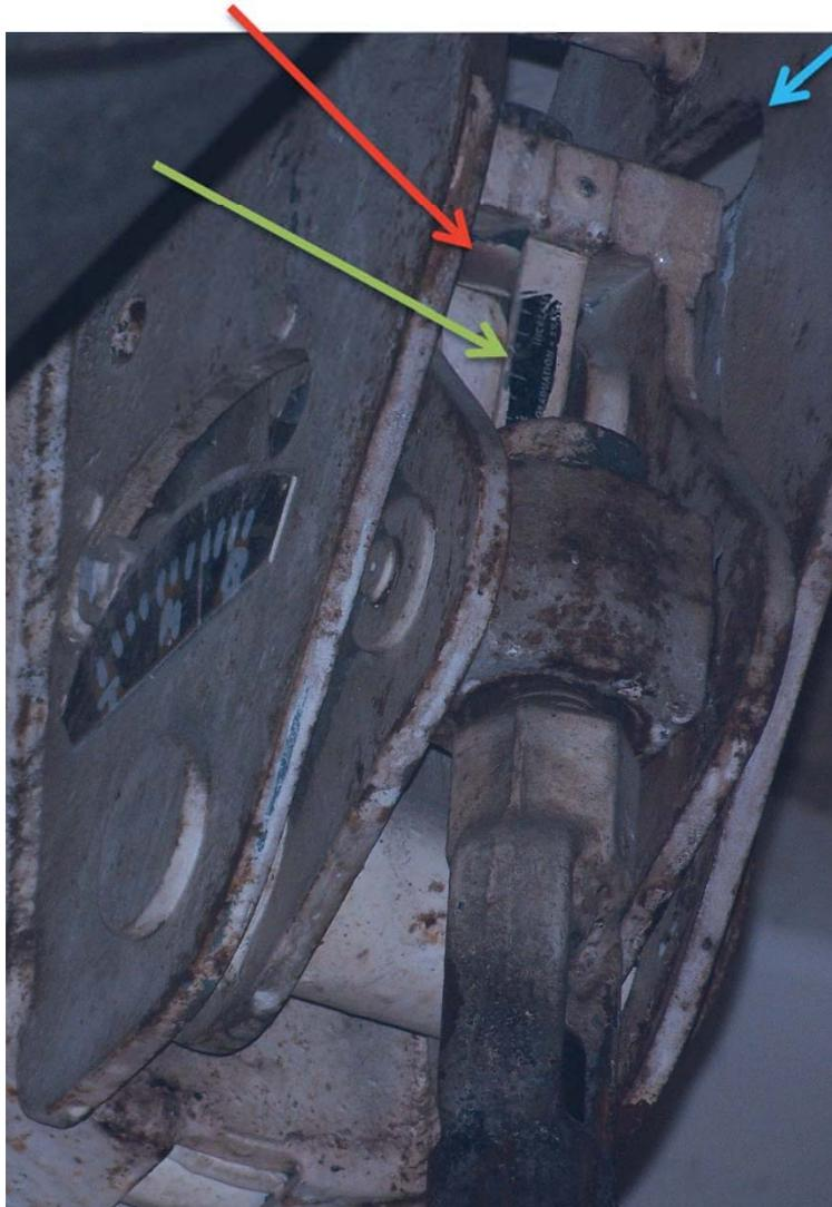
Another style constant support load scale shown by green arrow. Load bolt is behind scale, red arrow, and accessible only through the slot on the back side of the can, blue arrow.
