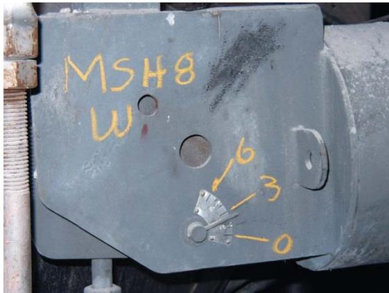
An old constant support can with a travel scale from 0 to 6. The indicator is a pin that can easily break off. It is recommended to paint the scale and scale numbers on a can when it is difficult to read or unusual. This will provide more consistency in later observations.
