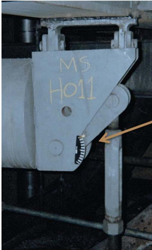
Another manufacturer's constant support travel scale. The indicator is just a piece of metal attached to the lever arm, which is susceptible to bending or breaking off. Note the scale has no numbers and observer has to visualize the direction of movement to assure which end of the travel scale is 0. In this case, as the rod goes down, the lever arm and indicator go down, so topped is 0 at the top of the scale and 10 is bottomed at the bottom of the scale. Reading in photo is 0.0.
