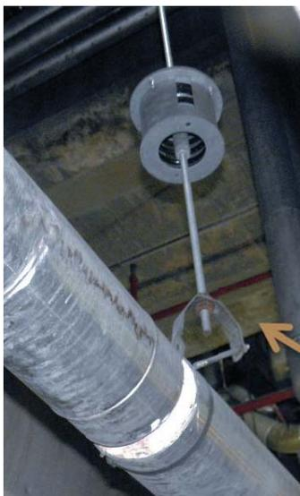
An example of Rule 1 is this variable spring hanger with the pipe clamp broken and completely disconnected from the pipe. The clamp should be on the pipe where the insulation is separated (white). The clamp was apparently on the pipe once, and is badly bent and above the pipe by 6”.
