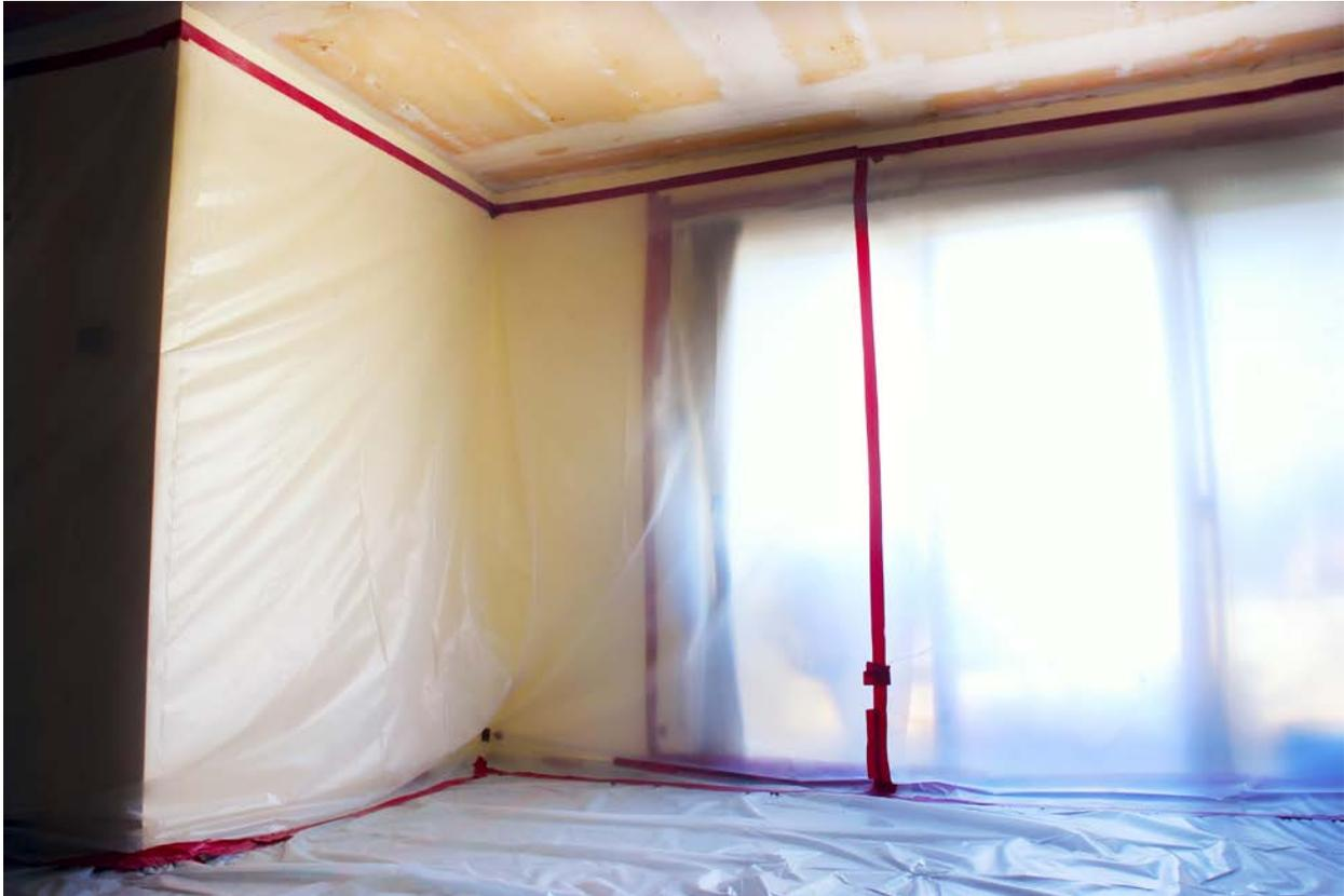
Picture No. 6 by [www.canstockphoto.com](http://www.canstockphoto.com) NPE with the polyethylene sheeting in place. Popcorn ceiling or similar coating appears to have already been abated.
