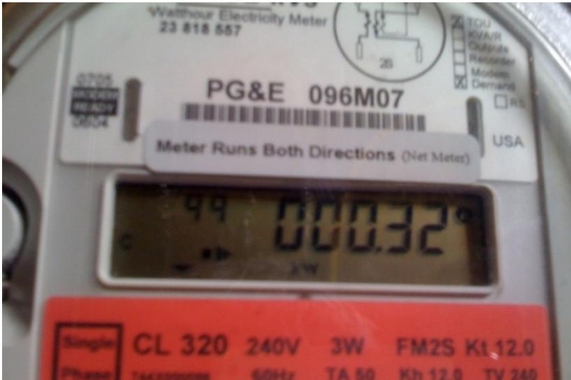
**Figure 20 Utility meter provided for Net Metering including an affixed label that reads “Meter Runs Both Directions (Net Meter)”**
