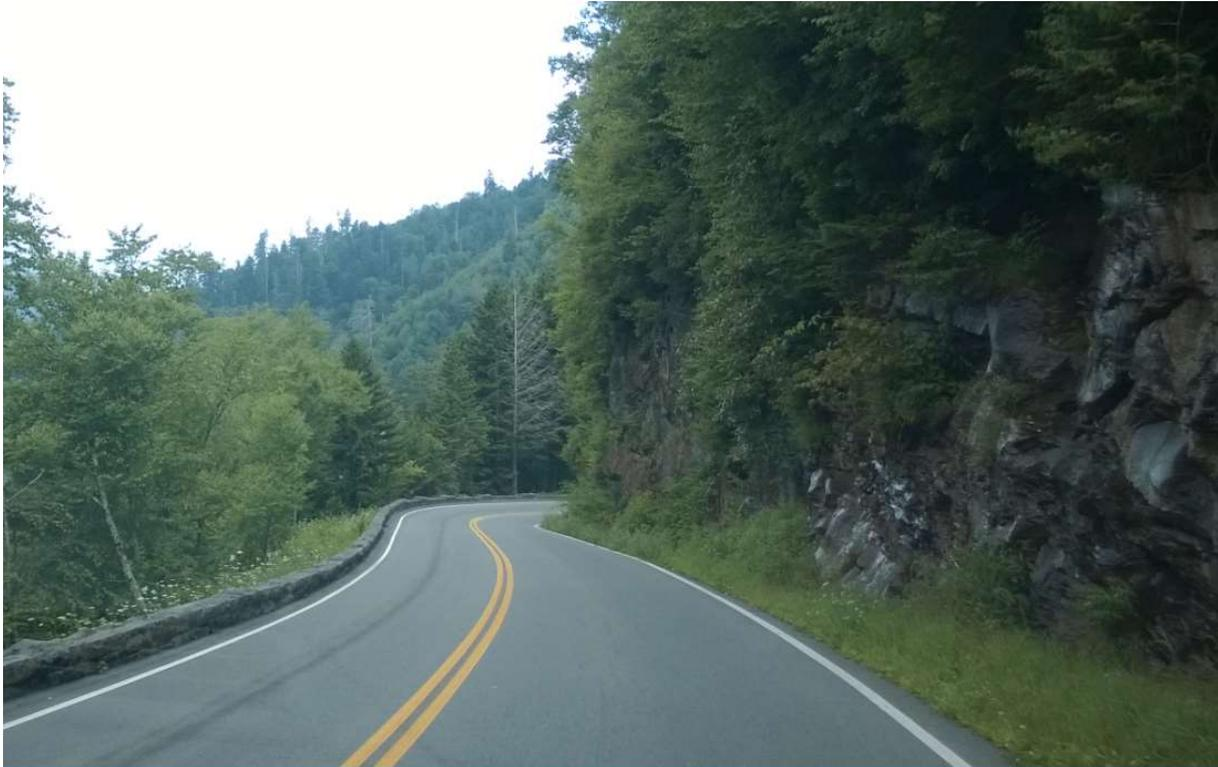
Figure 25. Horizontal curve with limited sight distance
