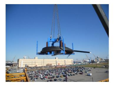
Strand Uncoilers – safely transport, protect, and facilitate installation of tensioning strands and prefabricated tendon bundles.
