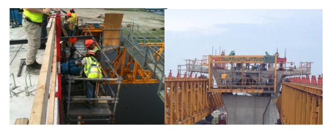
Stressing Platforms – Provide access and support for material installation and equipment use, some equipped with chain falls and trolleys for the hydraulic jacks
