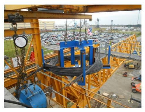
Ensure Strands are not Crossed, Install anchor plates and seat wedges on dead end of tendons, install anchor plates, wedges, and prepare hydraulic jacks for tensioning on live end of tendons.
