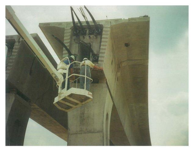
After the setting and joining of the segments of a span is complete, the post-tensioning operations will begin. Install permanent internal and external post-tensioning strand and rod longitudinally through the span. The number of strands per duct and the number of ducts per span will vary and a stressing sequence will be provided in order to transfer a uniform load. The strand is stressed using high strength hydraulic jacks. When the
