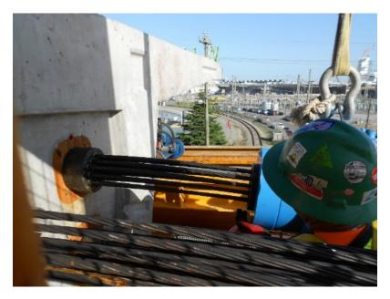
Pre-stressing Jack check – Jack and gauges will have been calibrated together, ensure the gauge corresponds to the correct jack and the calibrations are up to date and correct, verify service gauge with supplied master gauge. Visually inspect gauge and jack for wear and damage. Review Safety precautions. Cycle through jack operations to confirm it is working properly.
