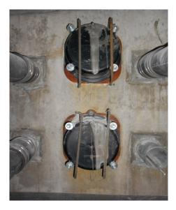
Reinforcing steel is drilled and epoxied into the segment face, a protective concrete block is cast around the plastic grout caps, and finally covered with and elastomeric moisture barrier.
