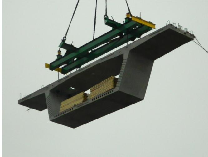
Crane lifting segments using picking frames and picking beams with anchors or sleeves
