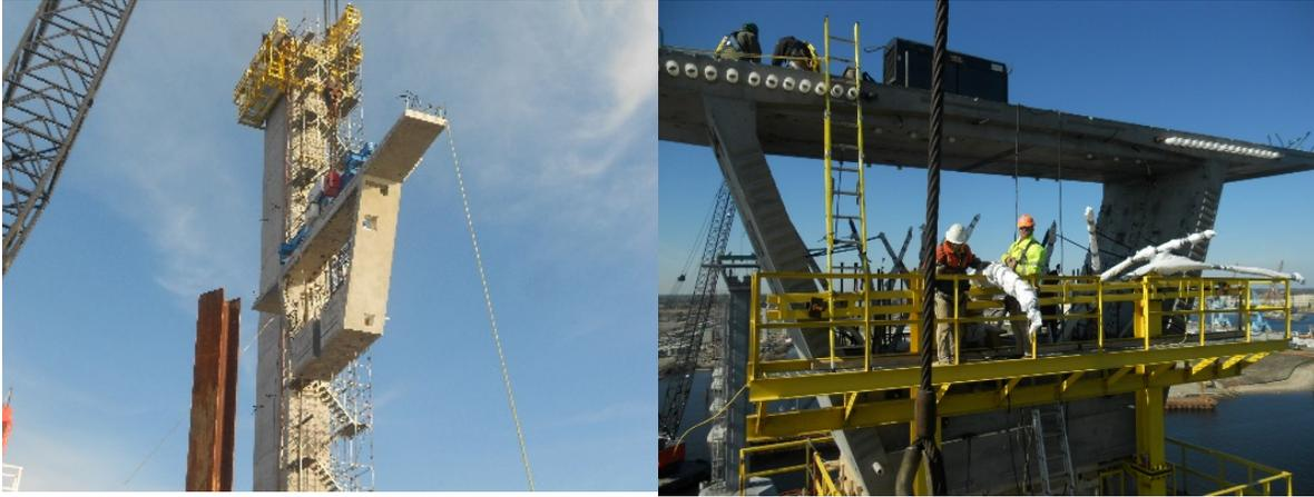
**Strongbacks:** Any segments requiring a closure pour that cannot be supported from below using shoring towers will need to be hung in place using strongbacks until the closure pour concrete is hardened and the post-tensioning steel is stressed. Strongbacks are steel beams which are anchored to the previously erected superstructure elements and hold the subsequent segment in a cantilevered position.
