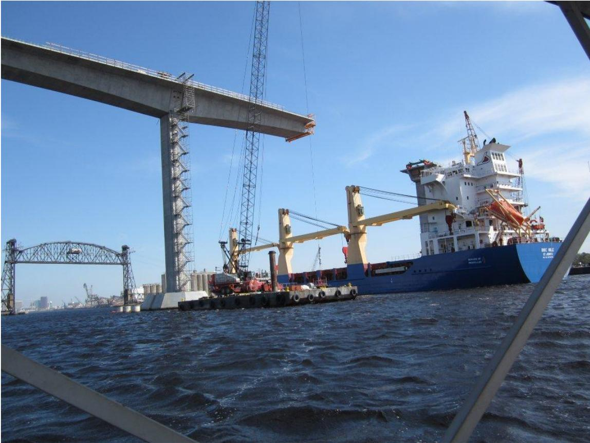
As with other segmental bridge erection methods, the typical segment erection is a repetitive process that gains efficiency with experience and scale.
