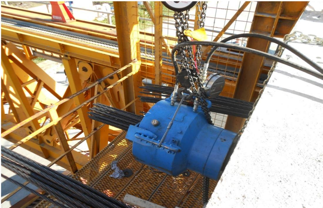
Elongations will be measured to ensure the stresses occurred over the entire length of the strand (a shortened elongation will mean the strand is pinched somewhere along its length and repairs may be necessary). The ducts are then pressure grouted to both
