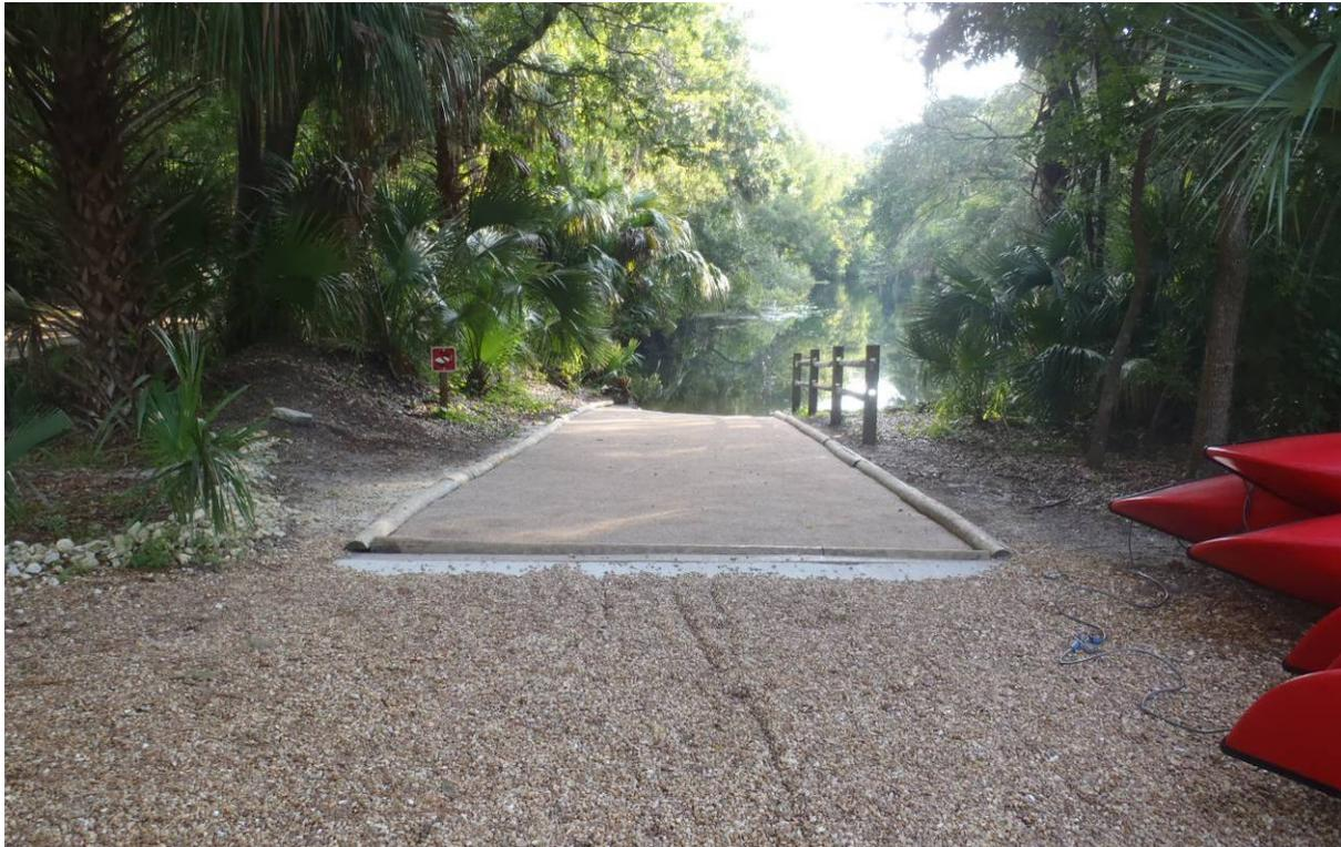
Figure 16 – Graveled approach to a NMB launch with a carpeted ramp at Silver River State Park
