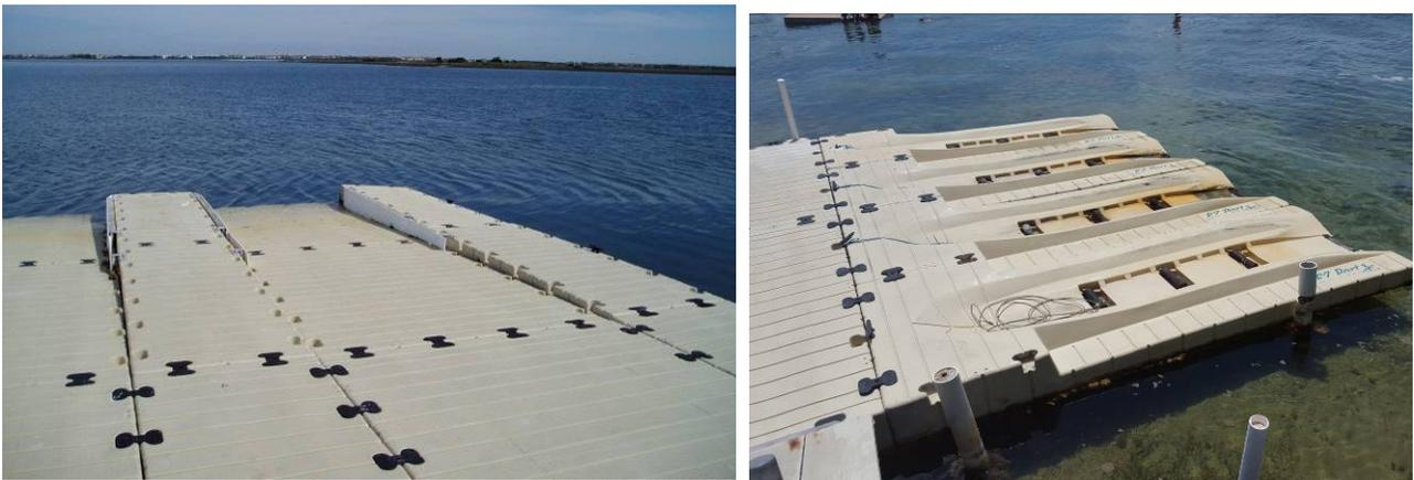
*Figure 23 – Floating docks with sloping ramps into the water for launching*
