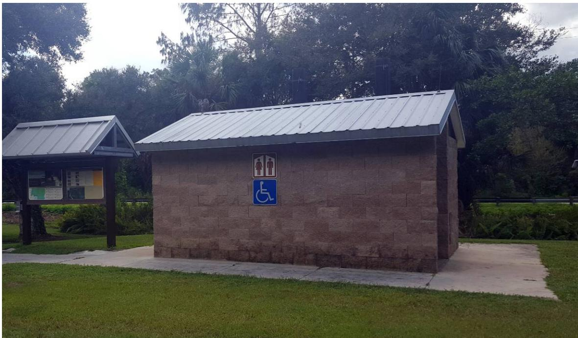
*Figure 24 – A CXT restroom facility without public water or sewer services available*
