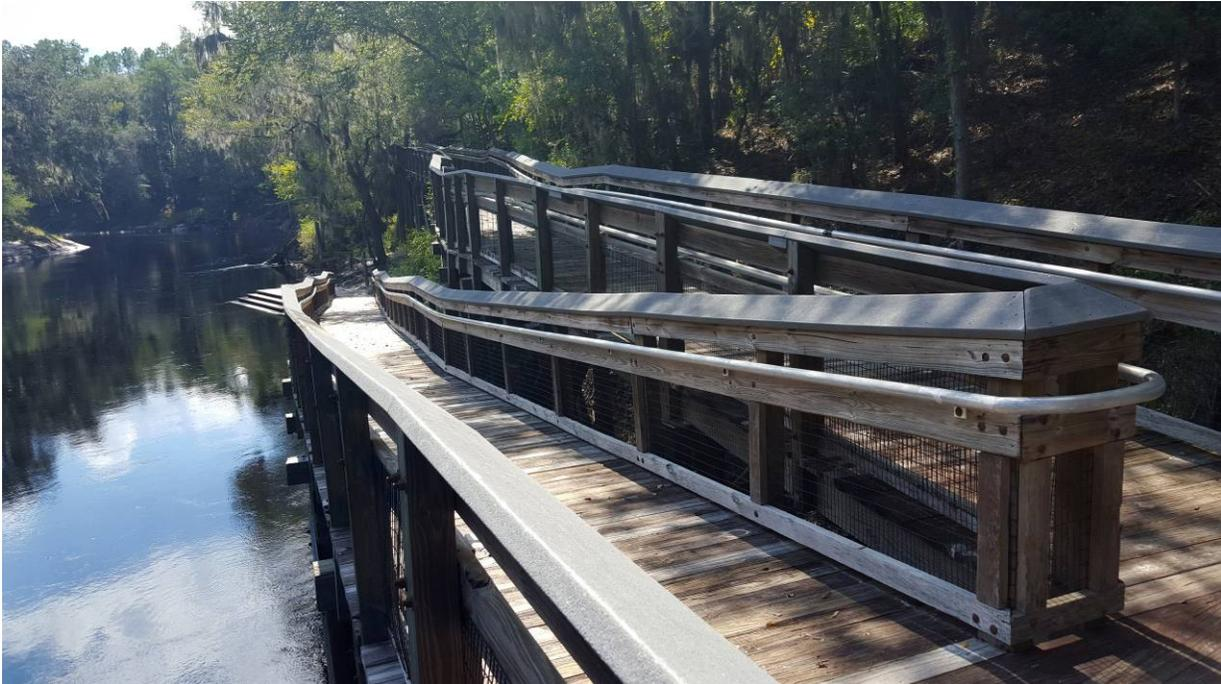
*Figure 29 – ADA accessible ramp from a high bluff that needs three switchbacks to get access to the water on the Suwannee River.*
