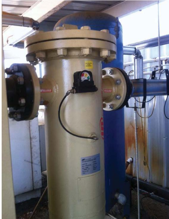
Photo 2: Particulate filter at dryer discharge.
