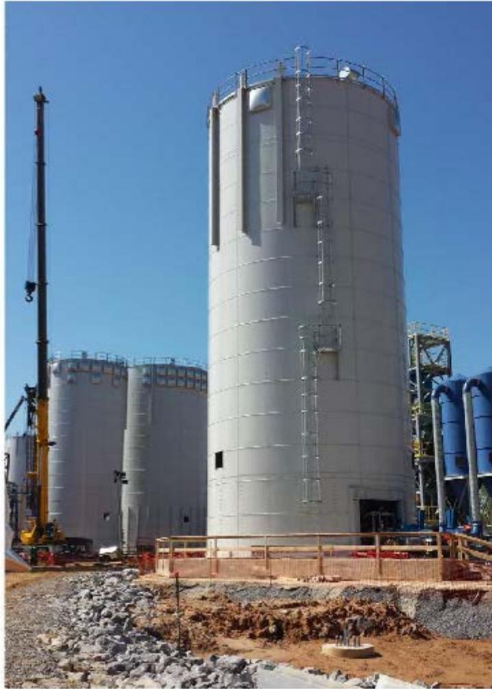
Figure 1: Silos under construction at a pellet plant. Note explosion panels in top walls. The columns extending part way down from the top are to support loads from a feed conveyor that has not yet been installed.
