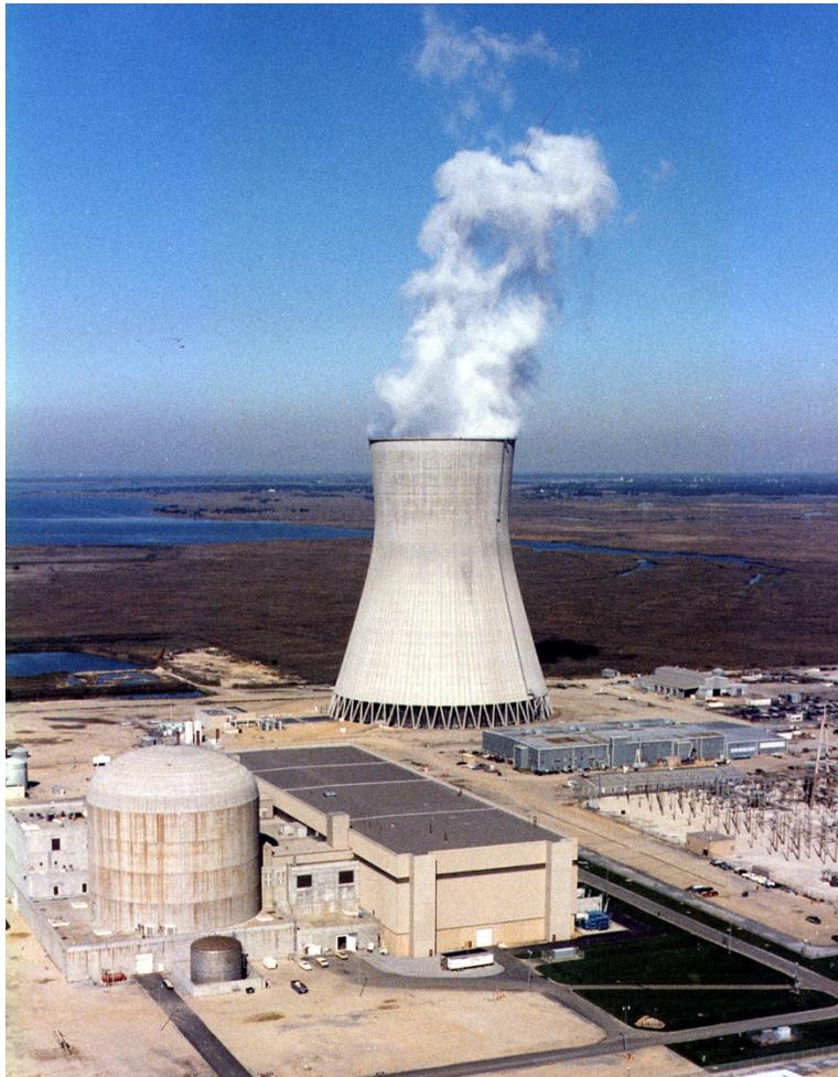
Figure 8: Natural Draft Cooling Tower at Power Generation Plant
