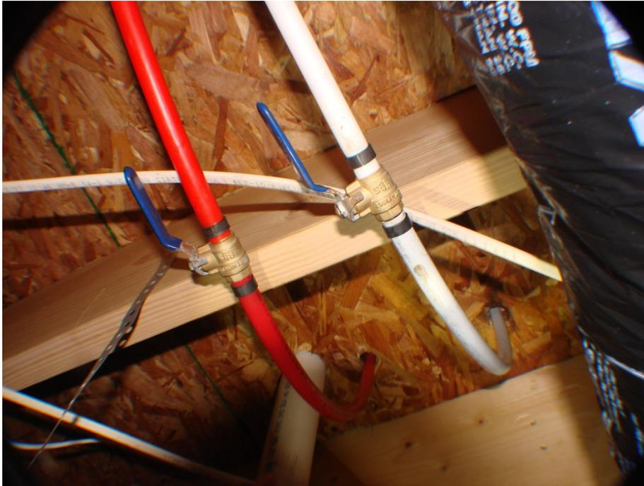
Photo #10 -- This is PEX tubing. If colors are used, red means hot, and blue means cold. However, coloration is not required by code and all piping can be white or clear. There are very few issues with PEX.
