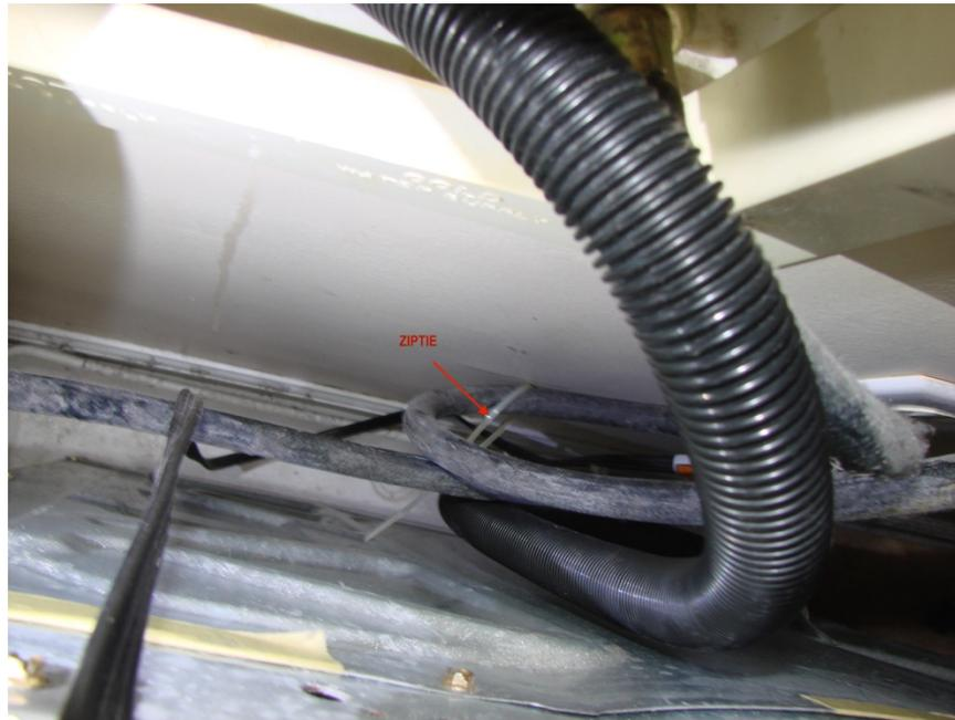
Photo #67 – The installer put a zip tie on the discharge hose but it failed and the hose popped out of the standpipe.
