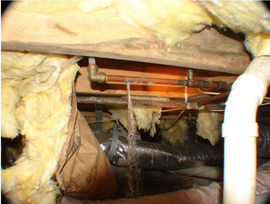
Photo #5 - The pinhole leak from pitting corrosion can lead to a significant leak if not detected quickly, as the pipe erodes due to the high velocity flow. The entire piping system in this house was affected by a water chemistry problem.
