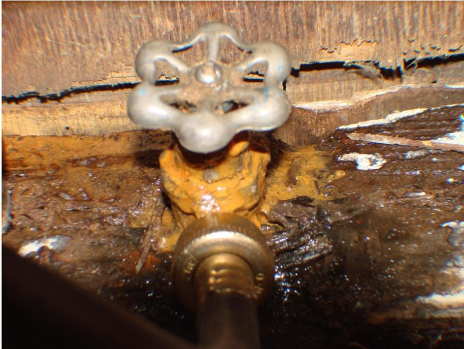
Photo #69 – The machine was not at fault for a long-ignored faucet leak.
