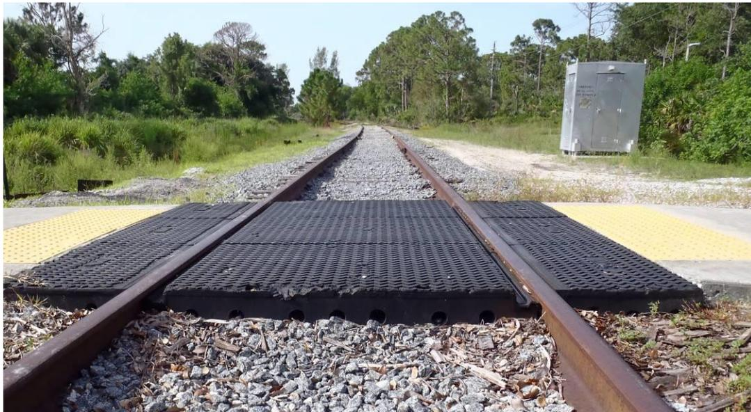
Figure 29 – A pedestrian rail crossing using synthetic materials
