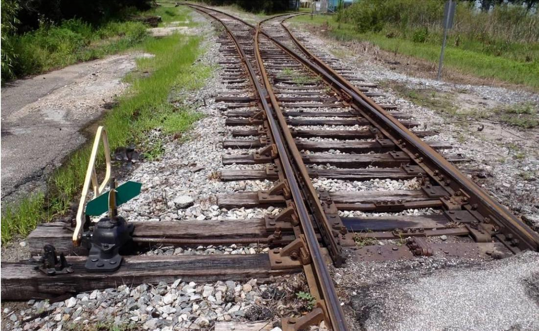
Figure 22 – A manual switch with a turnout for a customer's facility
