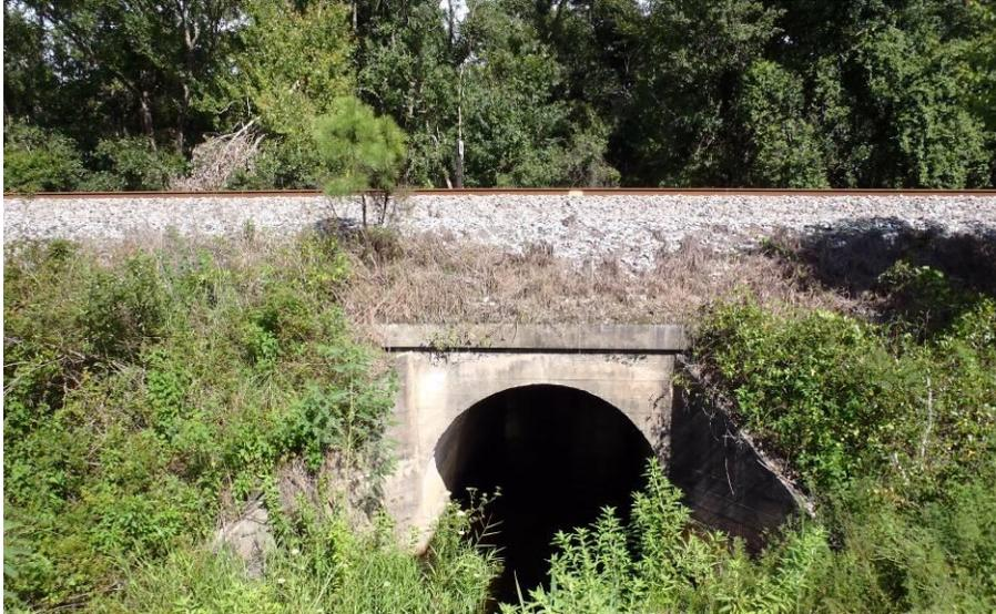
Figure 13 – Rail drainage system using a round culvert
