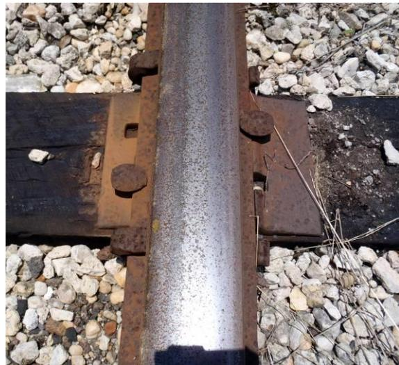
Figure 9 – An installed Tie Plate
