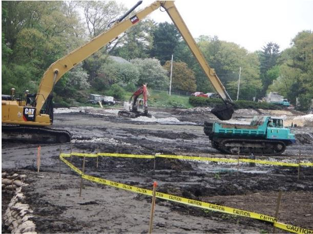
The Contractor should be responsible for the construction, protection and maintenance of temporary stockpiles through the final disposal. The idea is that the Contractor will place stockpiled soils within the designated stockpile area, graded to shed water, and will cover the stockpiled soils prior to inclement weather and at the end of each work week with an impermeable barrier of a minimum six-mil-thick (0.006") black polyethylene cover
