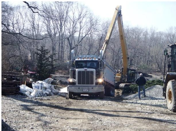
The contractor will need to ensure the material in the truck bed is covered and not draining water out of the back. Some water leaking may
