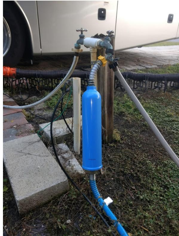
**Left:** A typical potable water connection on an RV
