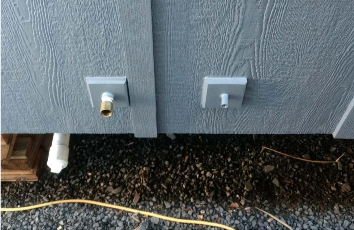
**From Left to Right: Gray water discharge connection for sink, potable water hose connection, potable cold water drain outlet used for winterization of this THOW**
