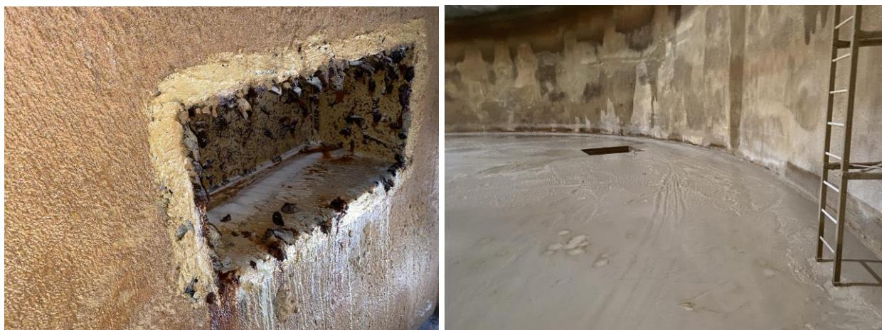
Figure 13: Examples of lime sludge found inside a ground storage tank.
