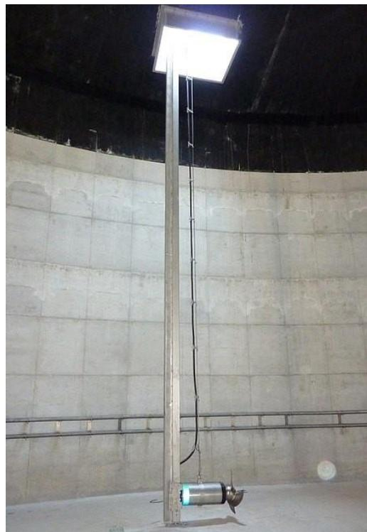
Figure 10: A rail-mounted submersible mixer which is removable from the hatch above.
