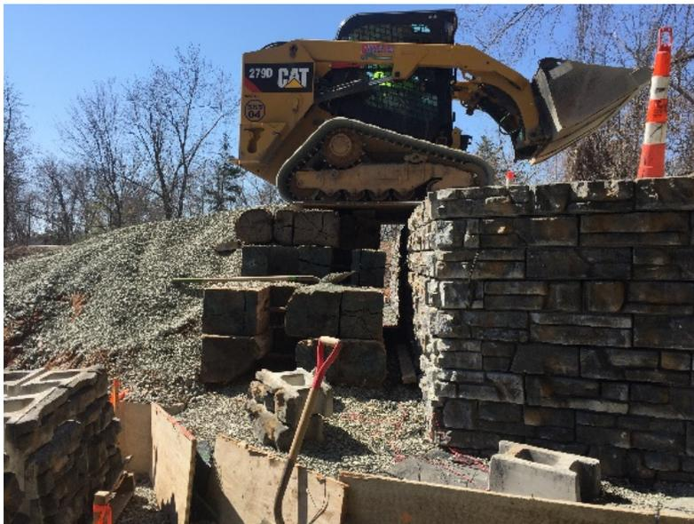
Rubber Tracked Skid Steer: Low clearance and maneuverable. For delivery of materials and spreading and grading aggregates. The low profile is helpful on bridge reconstruction projects. Rubber Tracks allow for load distribution on and movement on loose graded No. 8 & 67 aggregate.
