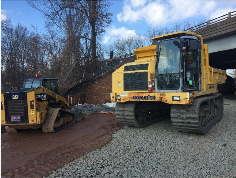
Tracked 360-degree Rotating Dumps: For restricted access bridge reconstruction projects, the 360-degree operation eliminates backing on long distances. Faster hauling and disposing of excavated material and delivery of backfill material. Tracks allow better load distribution and maneuverability in tight quarters.
