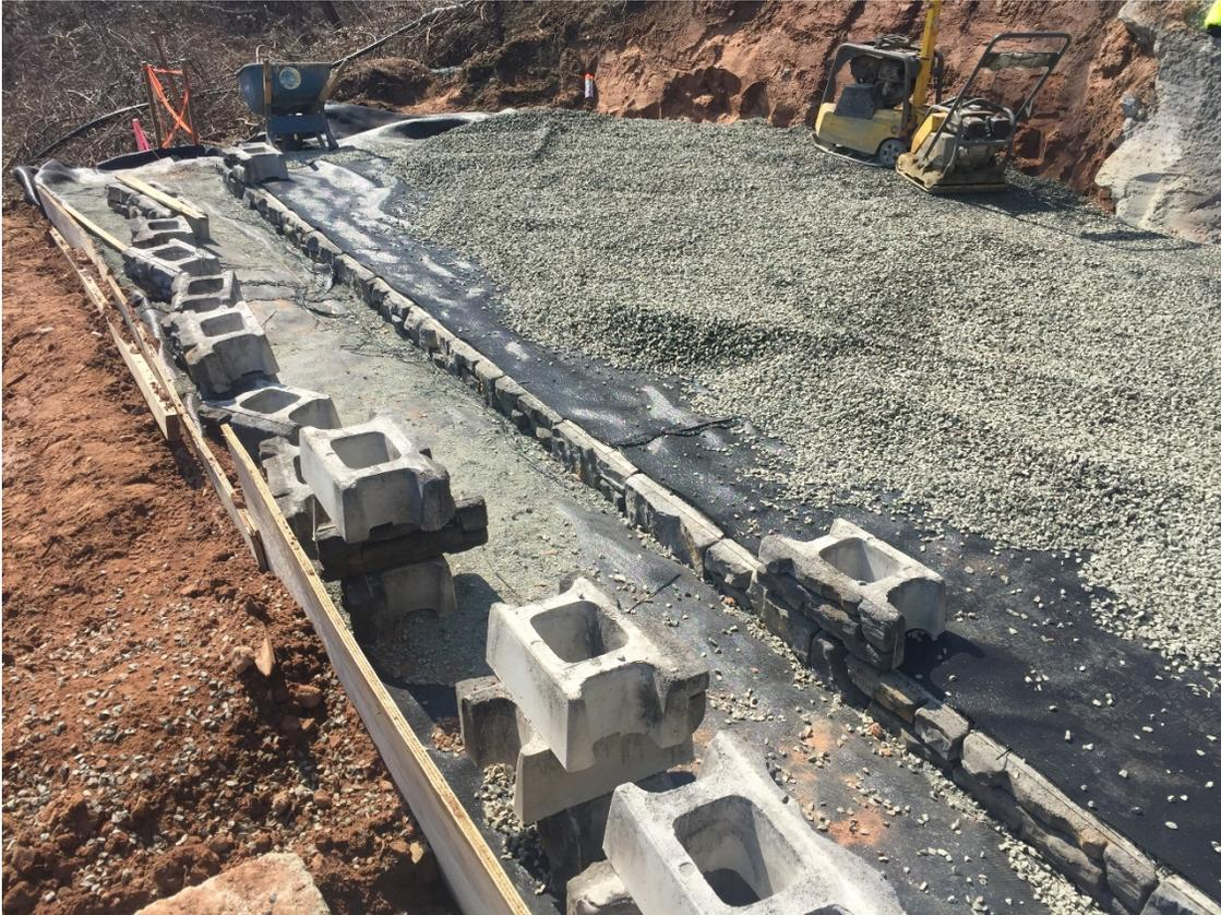
Regardless, any overlap at the CMU must be trimmed to avoid varying fabric thickness under the blocks which will cause instability. Place aggregate backfill in a constant direction making sure not to shift the geotextile fabric and cause wrinkles or tears. Stagger seams by a minimum of 2 feet with each successive lift of aggregate/geotextile backfill.
