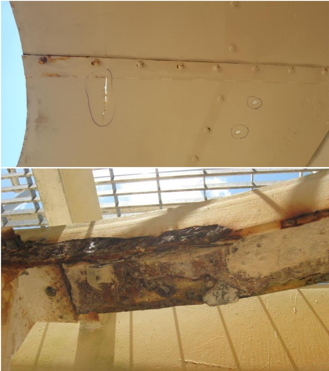
Figure 15: Solids contact clarifier with holes in the hood plates (top) and significant corrosion on the compression ring angles (bottom). These problems cannot be seen from the walkway, highlighting the need for an interior inspection.
