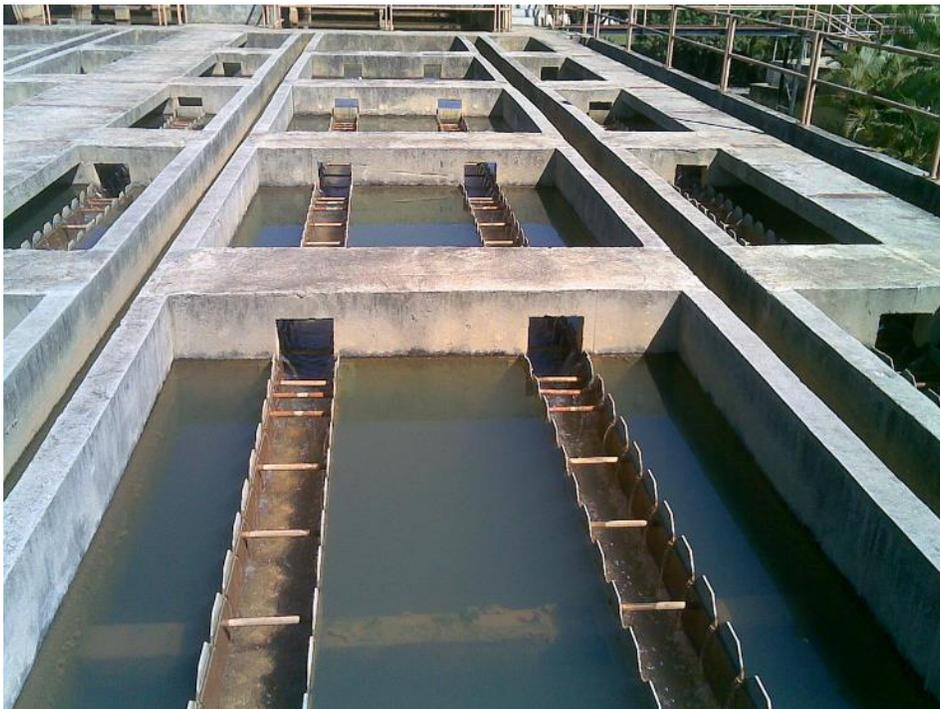
Figure 7: Rectangular clarifiers with effluent troughs.
