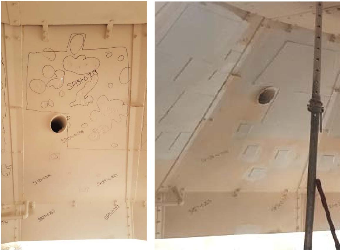
Figure 43: On left: Plate with thin areas delineated with black circles and the extents of the reinforcing areas drawn in black lines.
