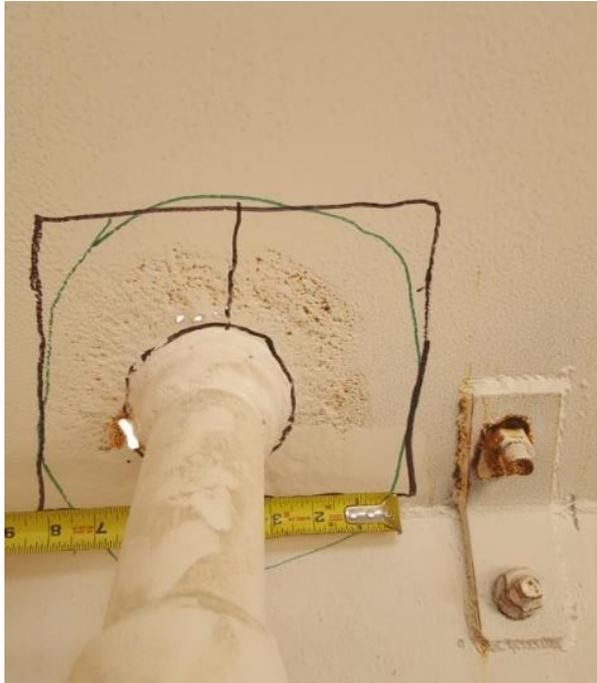
Figure 42: Thin steel discovered near a pipe penetration.
