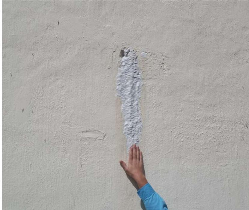
Figure 21: Example of efflorescence on the outside of a tank wall. Efflorescence is from soluble salts in the concrete being brought to the surface from passing water, thus indicating there is a slow leak in the area.
