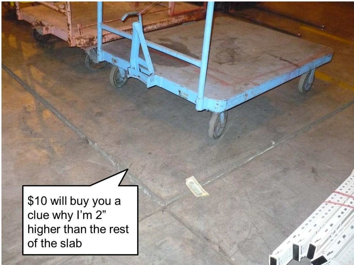
Fig. 7 - Slab distress at settling soil
