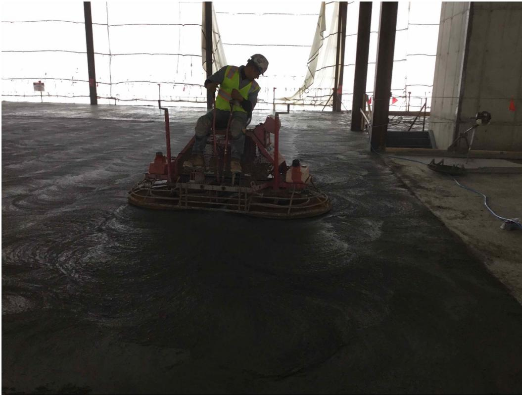
Fig. 18 - Riding power trowel with steel blades
