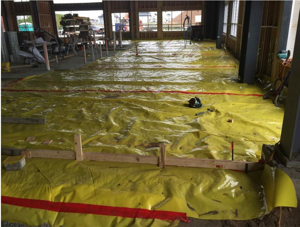
Fig. 9 - Vapor barrier
