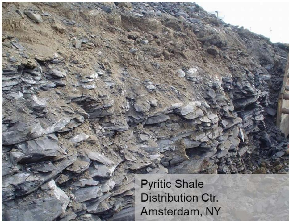
Fig. 5 - Removal of expansive shale in preparation for foundations and slab-on-grade
