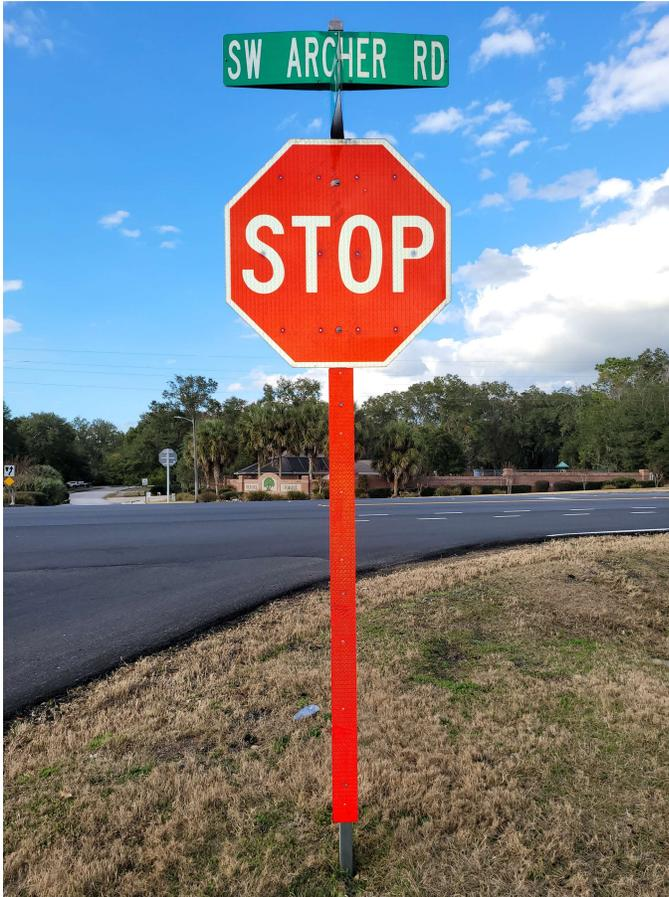
Figure 21. Reflective material on sign support
