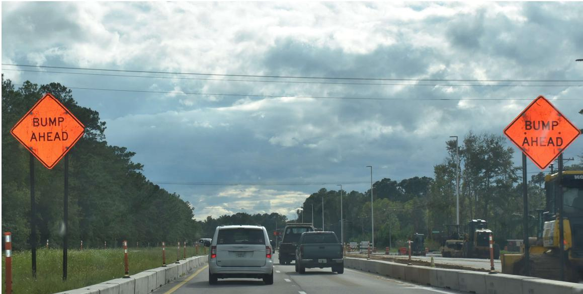
Figure 9. Placement of warning sign on both right and left to draw attention
