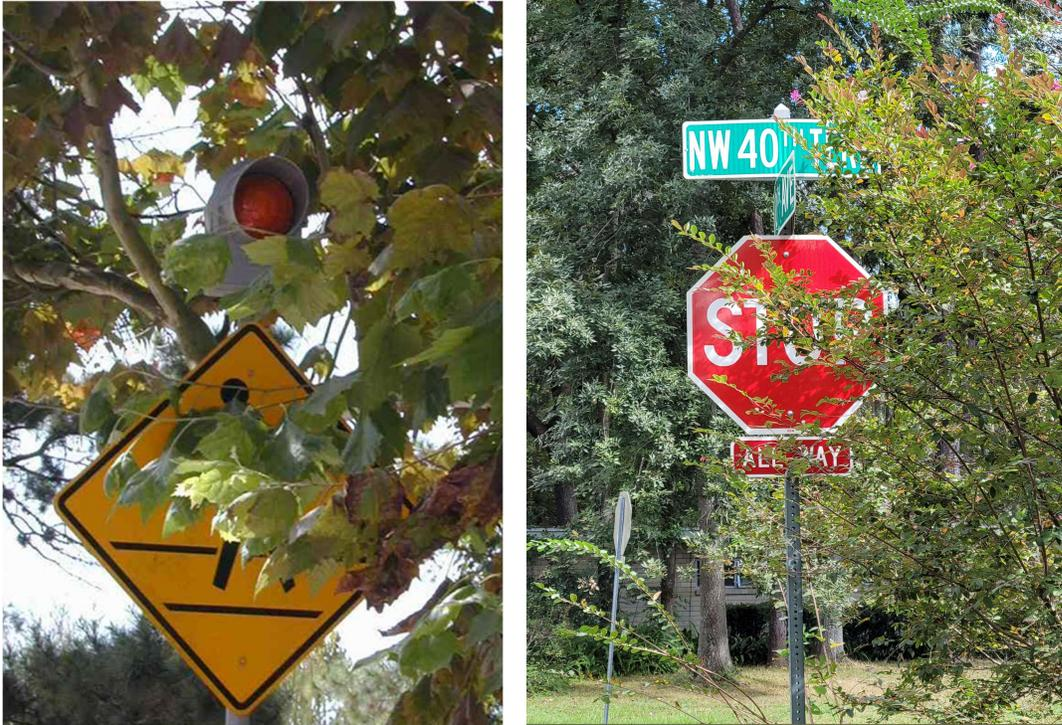
Figure 22. Sign maintenance needed
