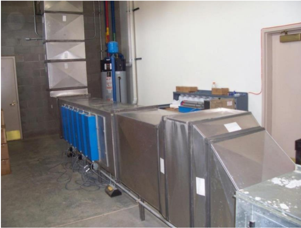
Figure 4: Example of an ionization odor control system. Inside the duct at the blue modules are a series of ion tubes.
