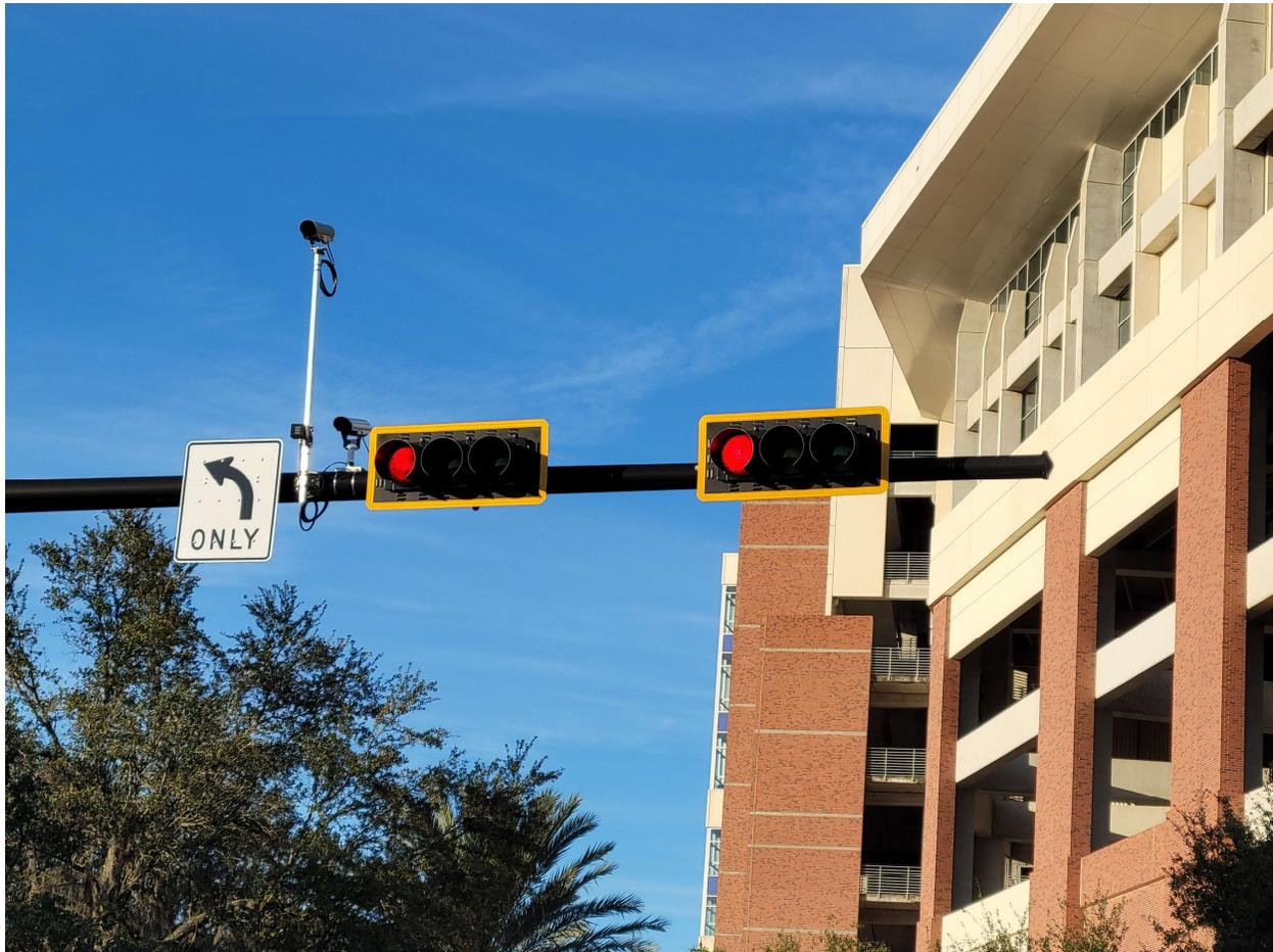
Figure 12. Signal head backplates with retroreflective strips
