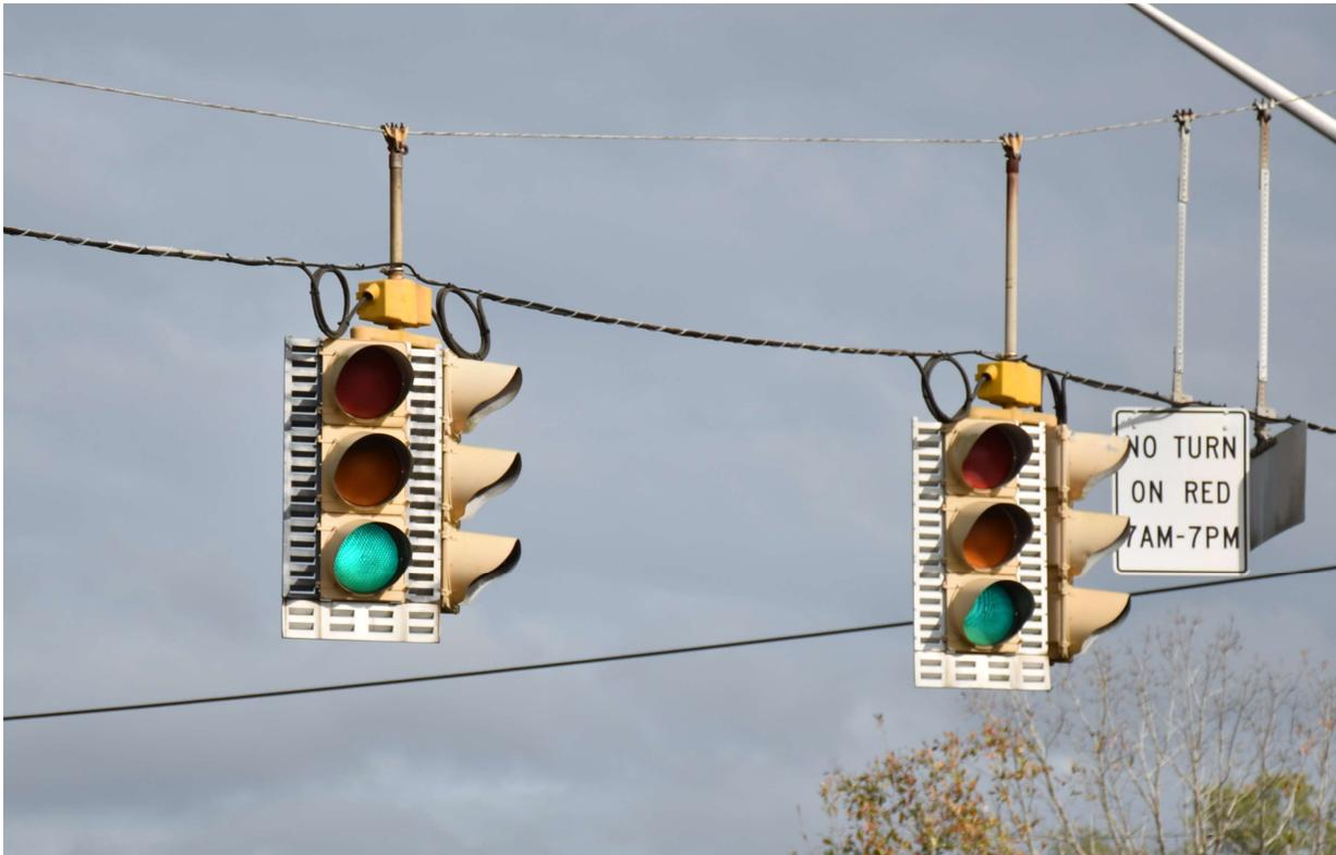
Figure 3. Faded paint on signal heads
