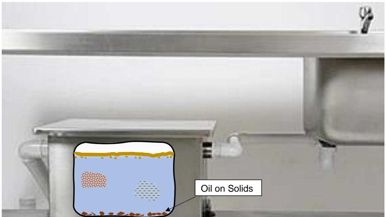
Figure 6: View inside a grease trap with oily solids at the bottom.
