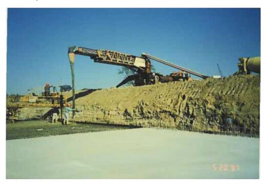
The last piece of equipment to cover is the Belt Conveyor Truck.
