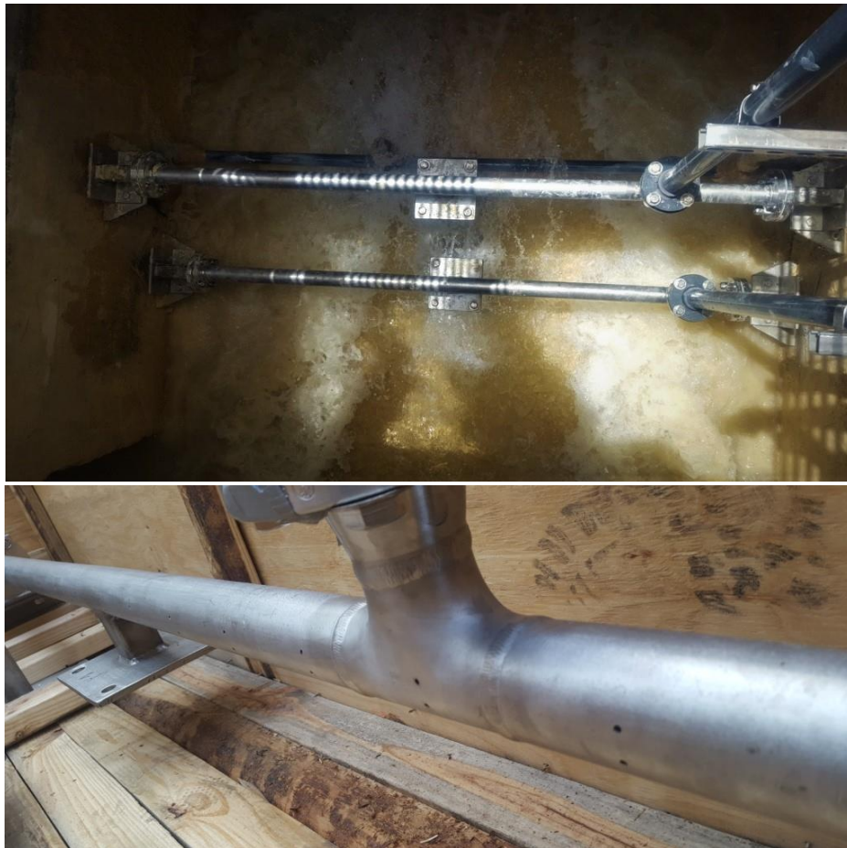
Figure 21: Examples of open channel diffusers.
