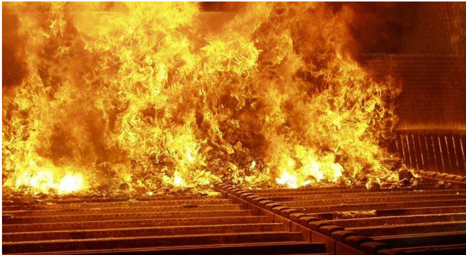
Figure 20: Solid waste combustion on a moving grate incinerator at a municipal waste-to-energy plant. Temperatures become high enough for the defluorination of PFAS.
