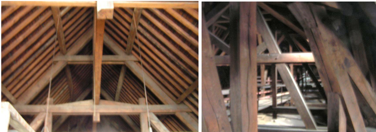
Figure 6: Views of "the forest" (attic) of the Notre-Dame Cathedral before the fire.
