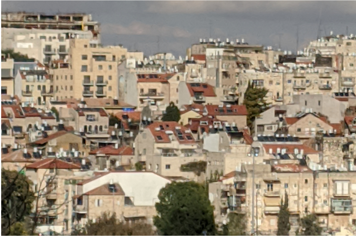
A plethora of solar heated water tanks and solar PV panels in Israel
