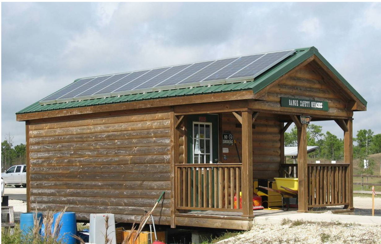
A small solar powered building
